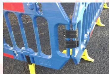
Some new road signs are self-ballasted and can withstand a Class C wind (19mph) (check manufactures data sheets for performance) **BUT** may still require fixing if there were strong persistent winds or heavy traffic caused movement of signs.
