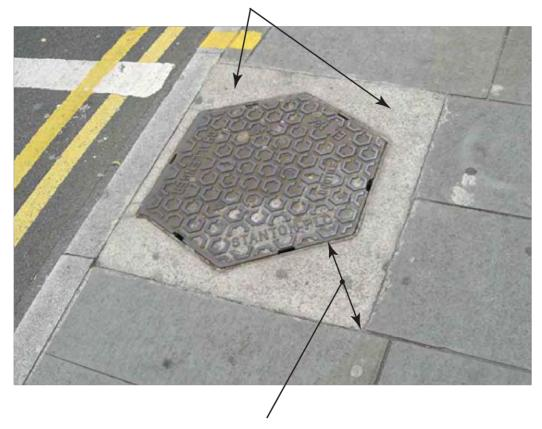
Maximum width of infill measured orthogonally from ironwork face increased to 200 mm to accommodate irregular shape
