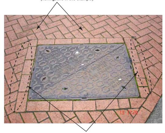
Use of larger blocks here creates acceptable loss of module pattern. This is preferred over using small angular blocks to maintain the pattern.
