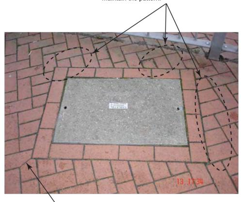
Use of larger cut blocks here leads to preferable arrangement of block pavers at the corners
