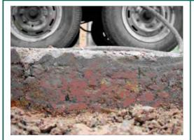
**EXAMPLE 3** DIRTY/DAMP EDGE CONDITIONS POOR BONDING [Weather: light rain]
