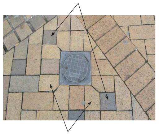
Use of larger cut blocks here creates acceptable loss of module pattern. This is preferred over using small angular blocks to maintain the pattern.
