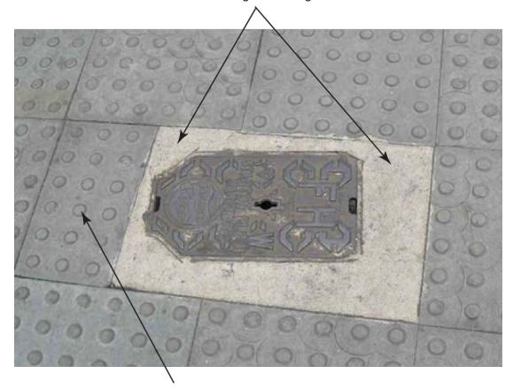
Using varying width infill limits cutting or trimming of modules
